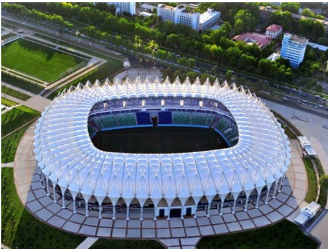
28-rasm. "Bunyodkor" stadionining tashqi ko‘rinishi (Toshkent)
